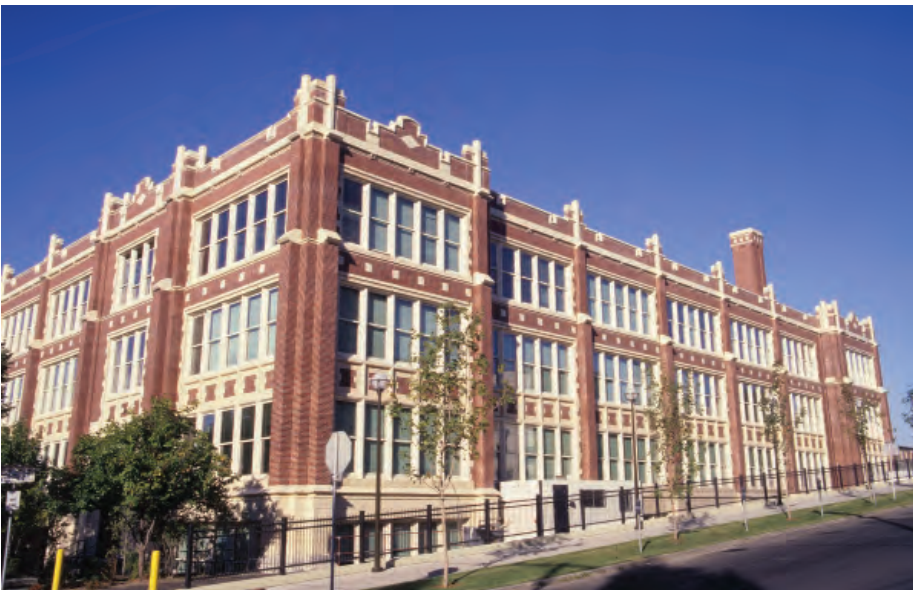
Built in 1912, Lewis and Clark High School in Spokane, Washington has been renovated to meet state-of-the-art standards.
